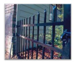
Anything attached to the house (decks, porches, fences and outbuildings) should be considered part of the house. These act as fuel bridges, particularly if constructed from flammable materials.
